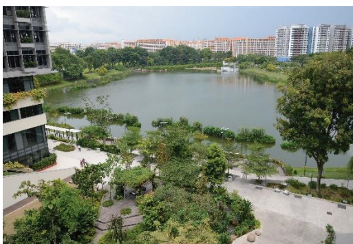
Figure 1.3.2 Retention Pond adjoining Khoo Teck Puat Hospital
